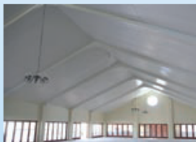
INFRA CEILINGS SET IN NEW BUILD CONGRESS CENTER BIG SIZE 120 CM x 300 CM
